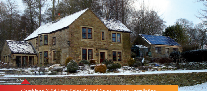
Combined 3.96 kWh Solar PV and Solar Thermal Installation, Longnor, Staffordshire.
